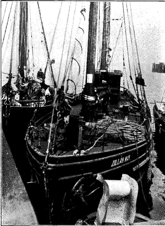
FIGURE 21.—Halibut vessel of older type, showing anchor cable. In foreground one of early chutes for setting gear. Seattle, 1915. Contrast with "Marmot" and "Pioneer."
